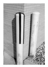
2. Slide the Post Guard over the bollard.
